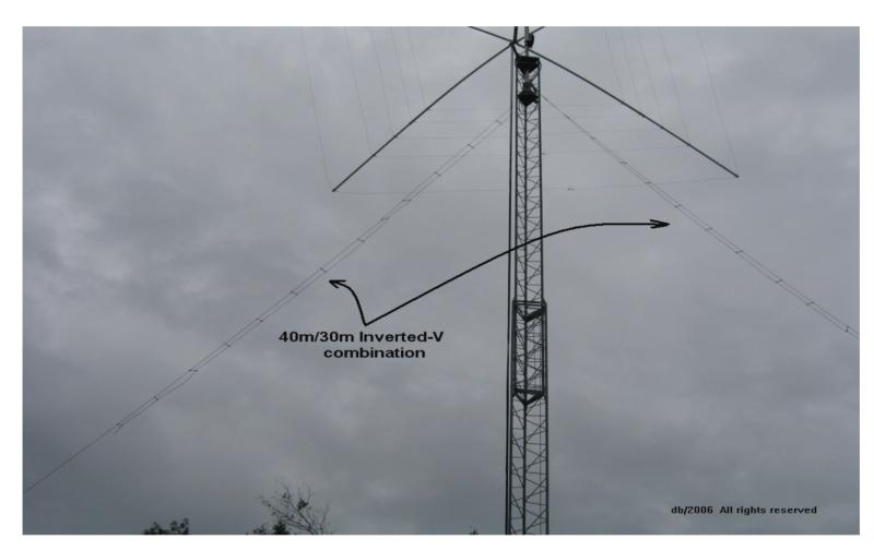
The 30m antenna hangs below the 40, suspended by 4" spacers made from readily available 3/8inch polybutylene water supply-line tubing, cut & drilled at each end to allow "threading" of the antenna wire through each. The coax feedline attaches to a commercial 1:1 balun, which also supports the antenna at the apex (a better angle view of the feedpoint may be seen below in the picture of the Quad).
