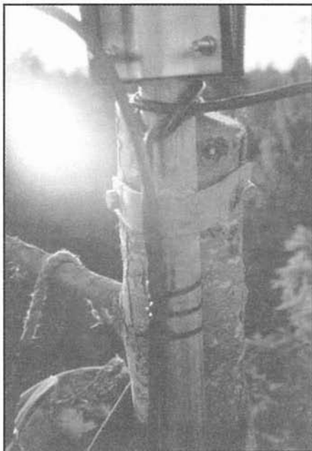
Photo 1: Mast mounted tree installation. Note horizontal brace for torque resistance.
