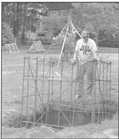
Photo 4: Lowering the rebar cage with a backhoe. Note nylon sling use.
