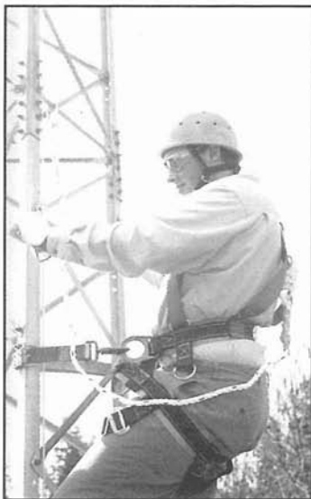
Photo 4: Our climber on the tower. His positioning lanyard is attached to the tower and the fall arrest lanyard is hooked to the tower above him.
