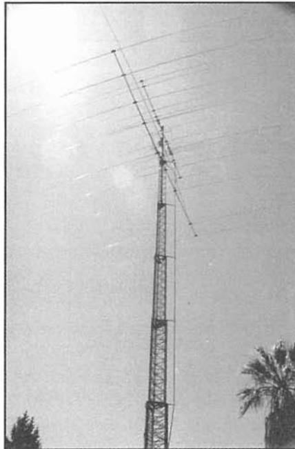
Photo 4: An impressively loaded and effective US Tower crank-up system owned by K6KR.
