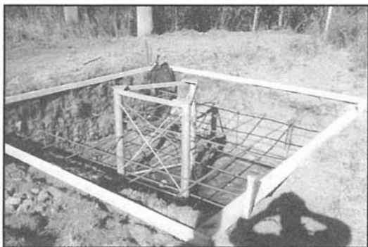
Photo 1: Typical self-supporting base with rebar, base section and ground level form.
