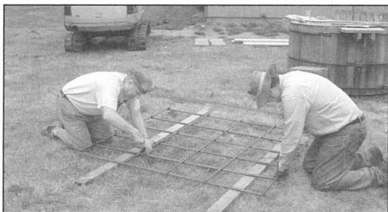
Photo 2: Building a rebar cage.
