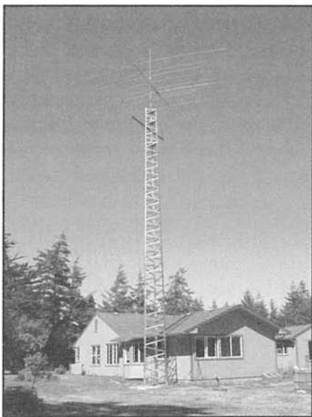
Photo 3: A Trylon Titan self-supporting tower in Bandon, OR. The proud owners are W7WWF and N7YYG.
