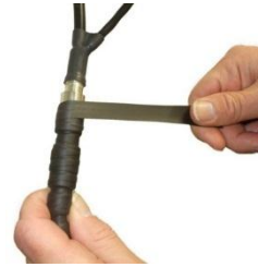
Stretching about 50% as you wrap Overwrap previous wrap by about 50%
