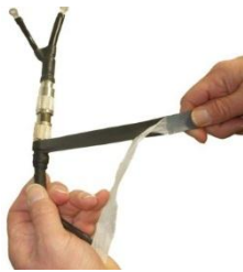
Wrapping peeled back as you wrap
