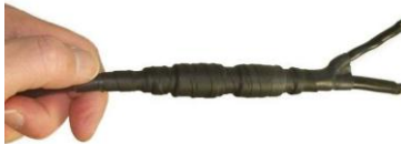
Completely wrapped with DXE-3M2155 Rubber Splicing Tape
