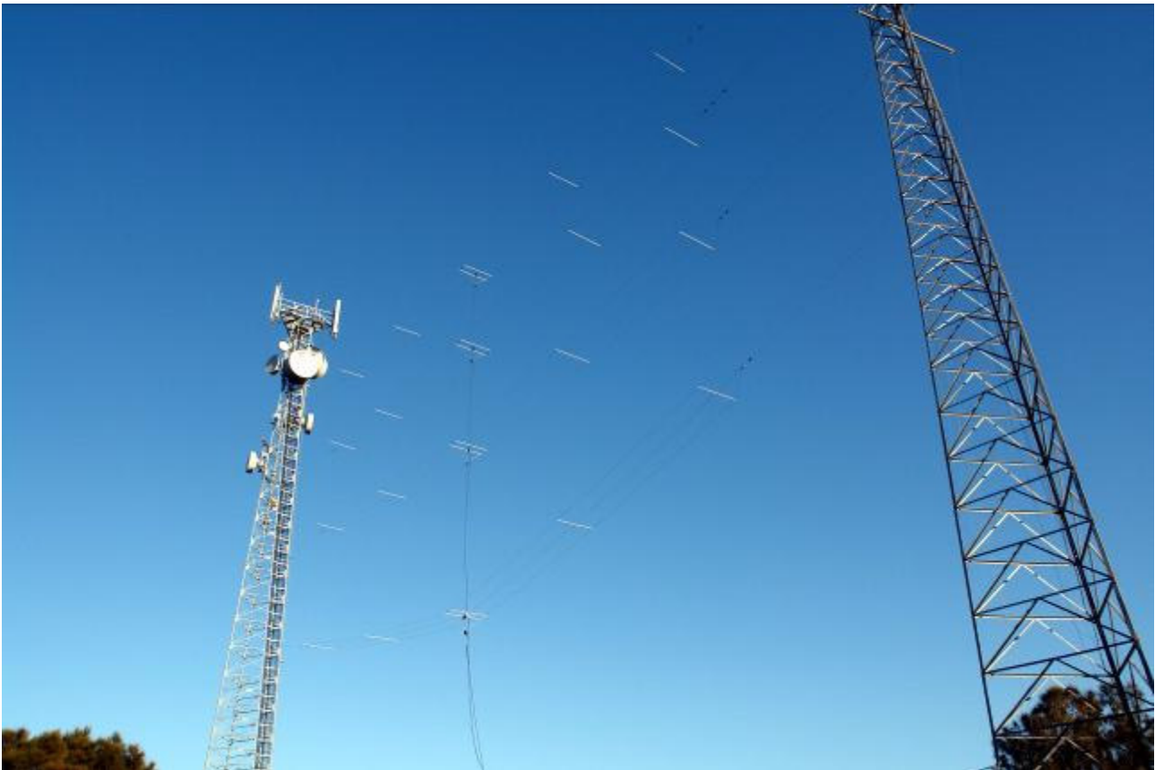
Bushcomm BBA100 and 1kw antennas used in a Barret communications facility—Courtesy of Bob Blumfield
