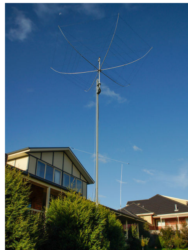
Free-standing hydraulic tilt-over metal pipe mast with rotatable "Hex beam".
