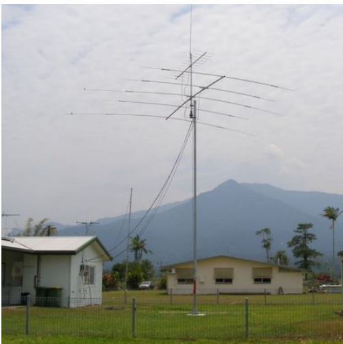
Tilt-over metal pipe mast with stacked rotatable Yagi beams and a VHF vertical.
