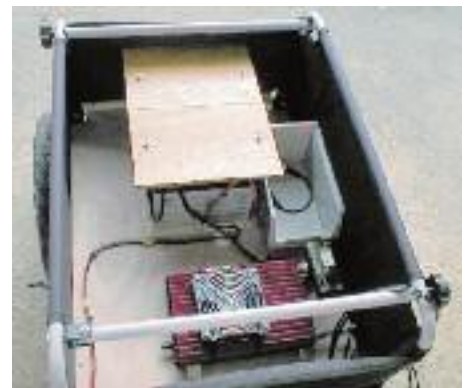
PHOTO 5: Inside the trailer there's a 250W amplifier and (under the wooden cover) 80AH of battery power.
